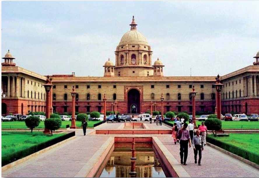
The Jewel in the Crown. The North Block of the Secretariat Building in New Delhi, a rare example of architectural glory in an Empire characterised by expedience rather than splendour. The building, housing the Ministry of Finance and the Home Ministry, was designed by the British architect Herbert Baker, working alongside the legendary Sir Edwin Lutyens.
